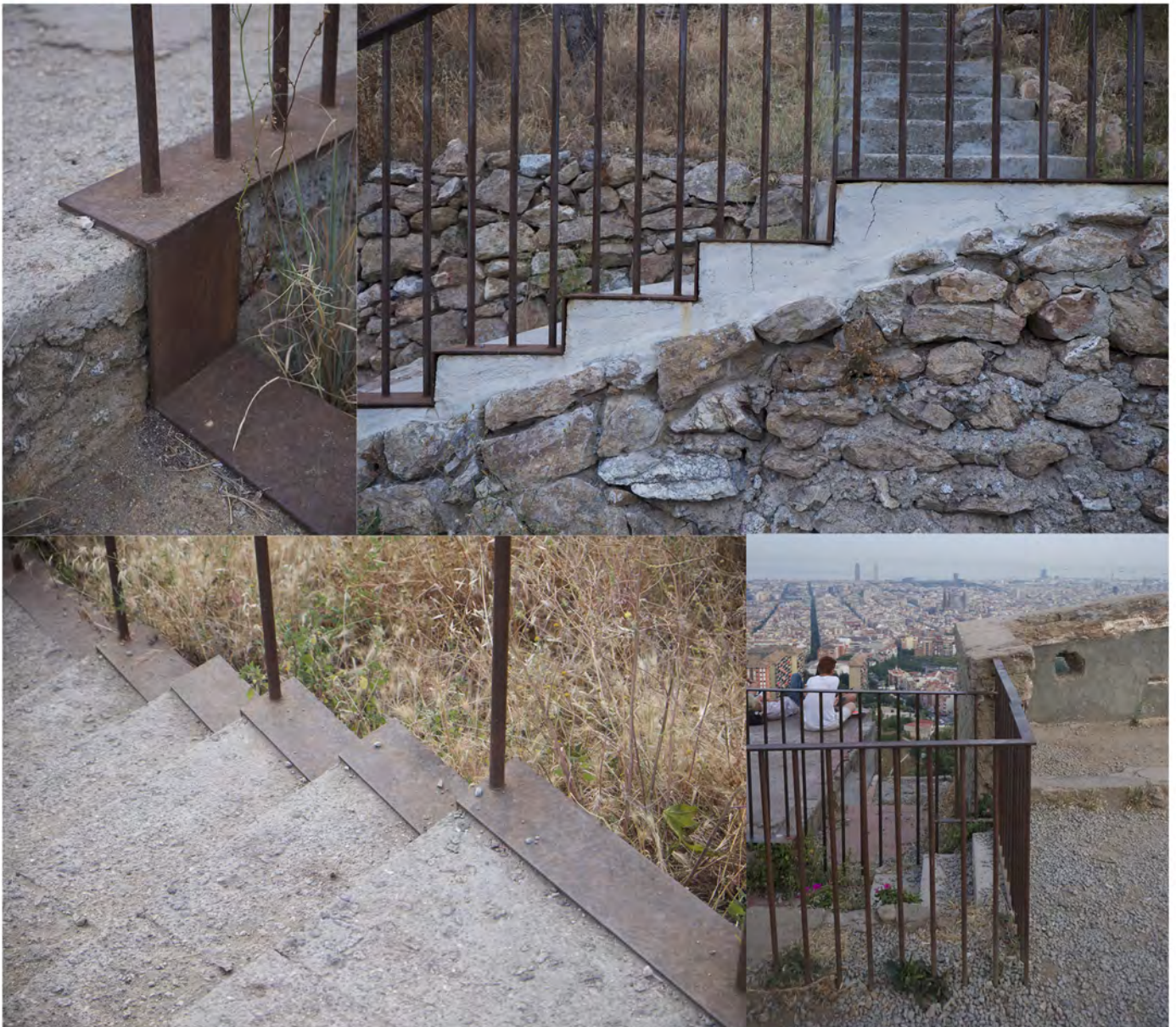
Turó de la Rovira, reinforcing steel and flat bar handrails and balustrade details. Photo: William John Maynard
