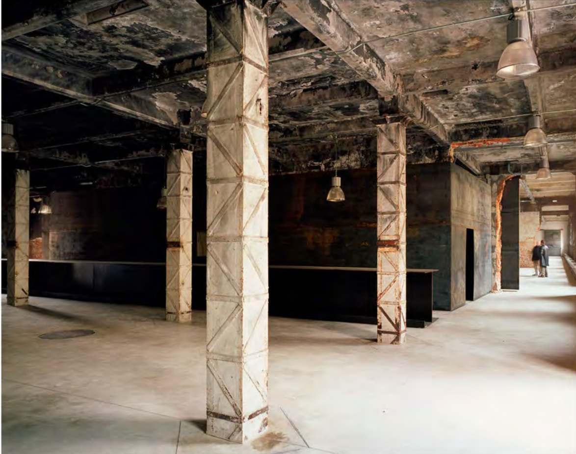
Nave 17c, interiors and entry ramp. Courtesy of Arturo Franco.
