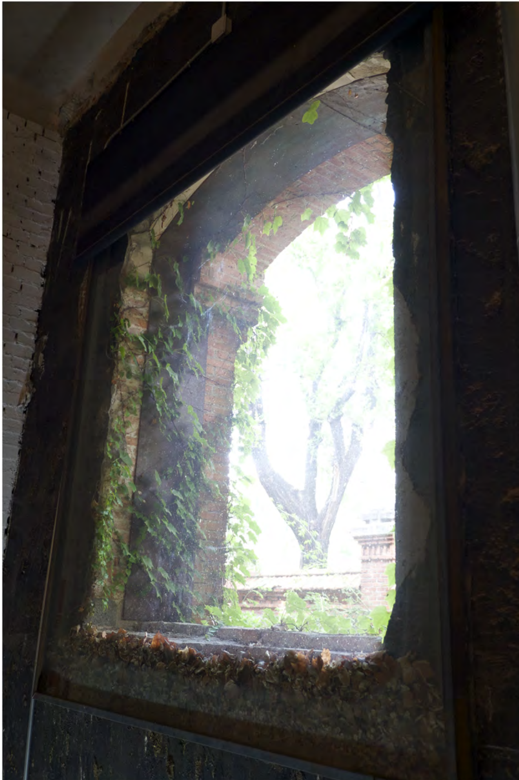
Internally fixed window assembly, Nave 17c, Arturo Franco. Photo by William John Maynard
